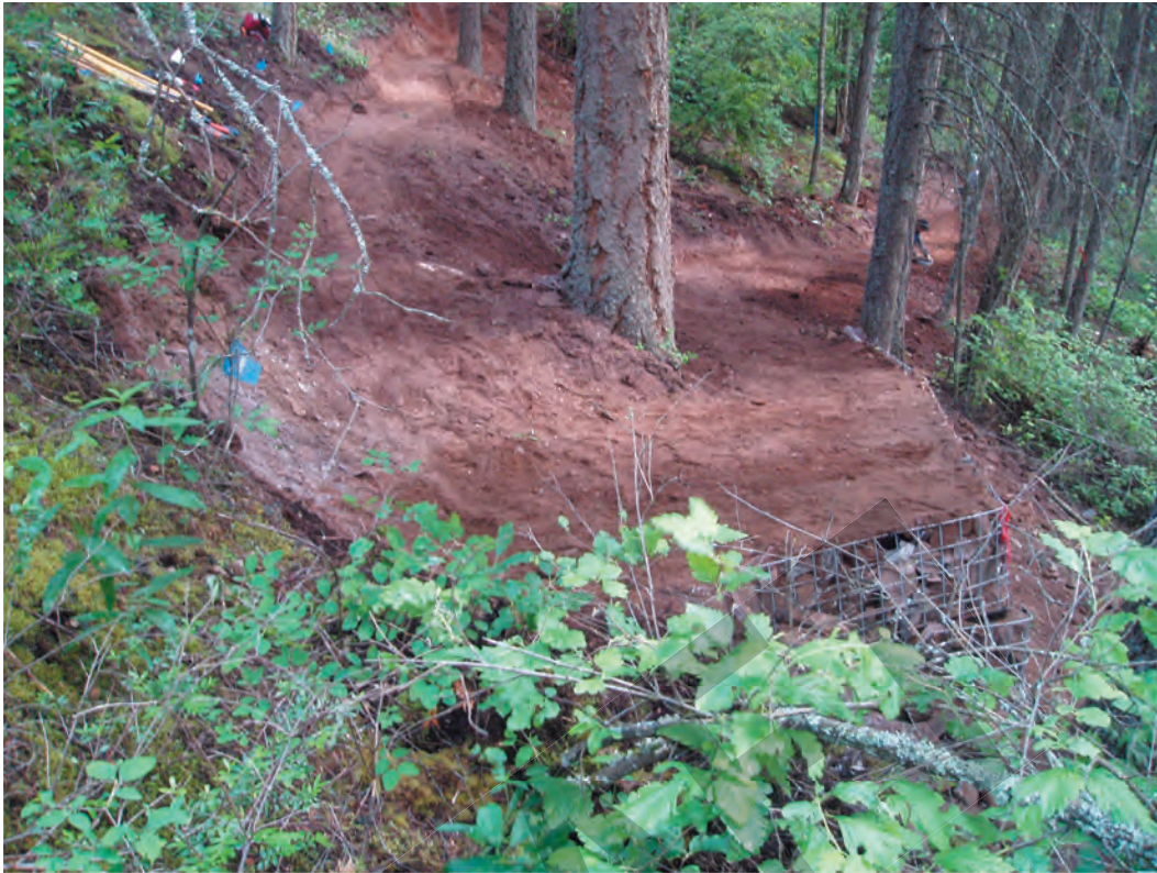
Anchors - Large Tree in switchback
