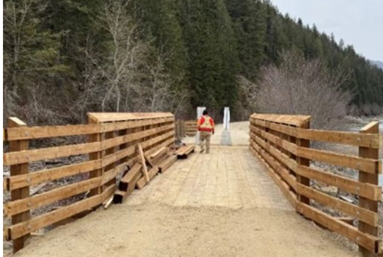
Shuswap North Okanagan Rail Trail Rosmond Lake Bridge
